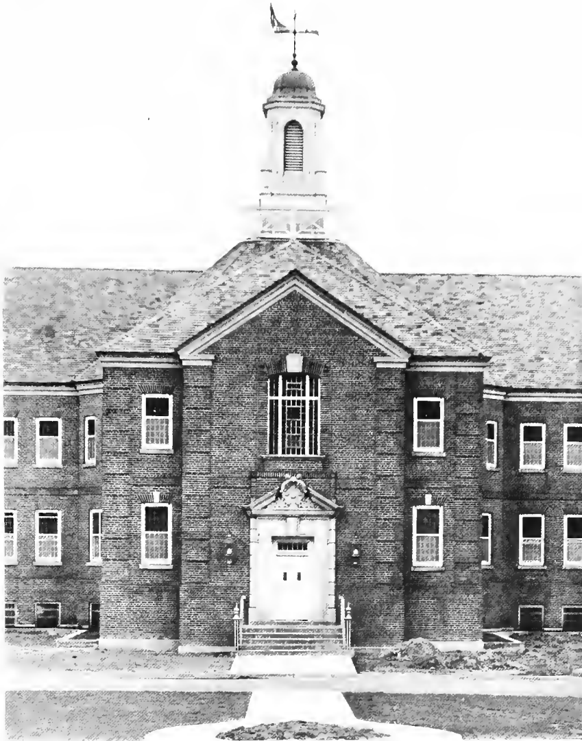
ENTRANCE DETAIL, NEWARK STATE SCHOOL
